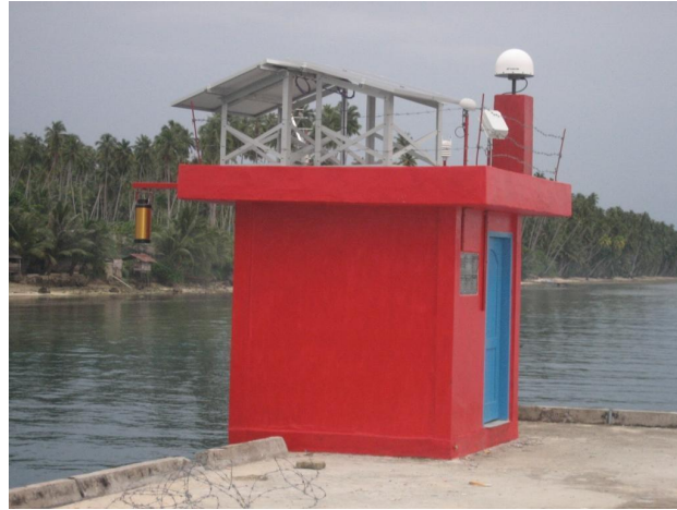
Figure 1: GNSS-controlled Tide Gauge (Tanahbala, Indonesia)
