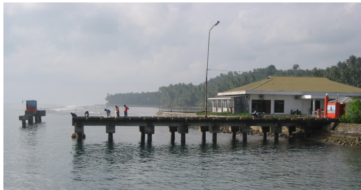
Figure 2: GNSS-controlled Tide Gauge (Telukdalam, Indonesia)
