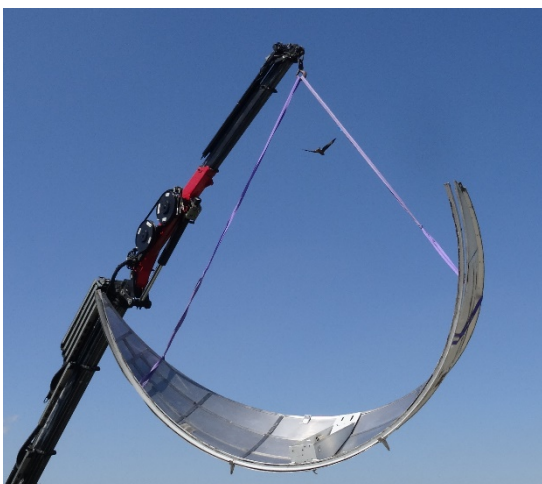
Figure 2: Dismounting of the old all-sky dome.
