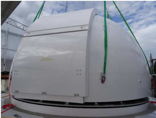
Figure 1: The new slit dome protecting the Zimmerwald Laser Ranging and Astrometry Telescope ZIMLAT was put in place on June 24, 2022.
